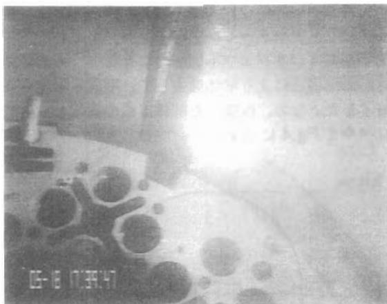
Photo 3 Cutting of Reactor Internal by Plasma Arc
