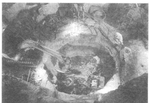
Photo 4 Mechanical crushing using a backhoe
