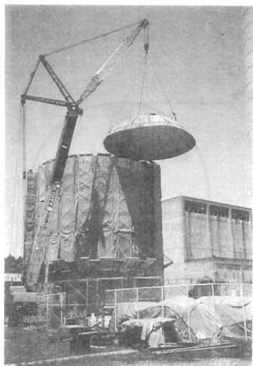
Photo 4 Removal of Outer Steel Plate
