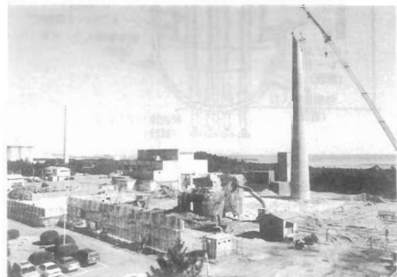
Photo 5 Demolition of Reactor Building and Stack
