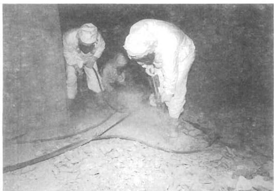
Photo 3 Removal of Embedded pipes using a Hand-Breaker
