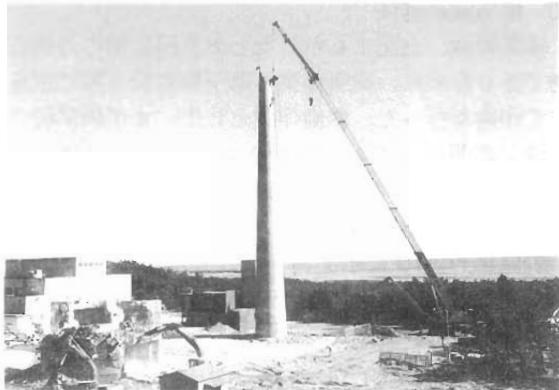
Photo 6 Demolition of Stack
